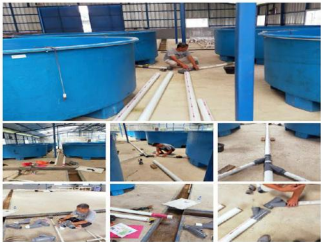
Fig 26: Installation process of outlet pipes and collector pipes in the broodstock and grow-out unit
