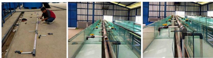
Fig 15: Installation of aquarium inlet pipes
