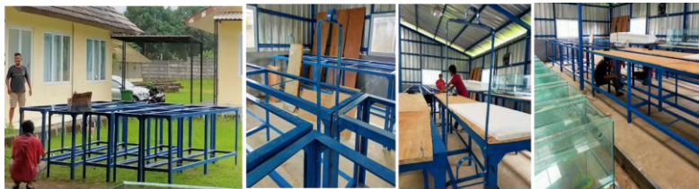
Fig 12: Arrangement of aquarium racks, including the installation of a base using plywood and Styrofoam
