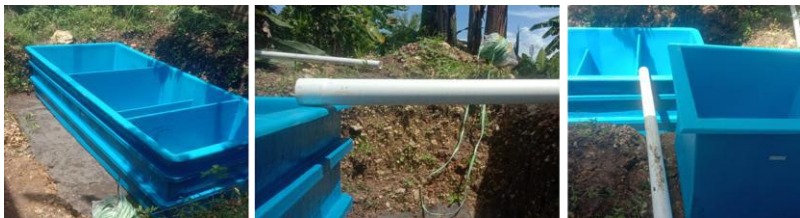
Fig 28: Installation of filter tank in the broodstock rearing unit
