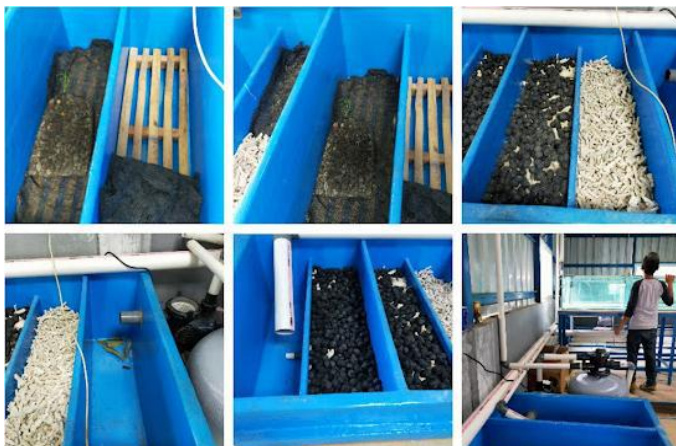
Fig 18: Installation of biofilter and connector pipes to the pump, sand filter, water storage and collector outlet pipes from the aquariums
